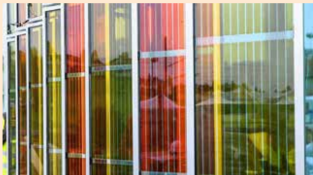
Detail of photovoltaic glazing
