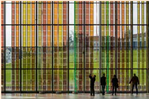
The new Swiss Tech Convention Center at EPFL (École polytechnique Fédérale de Lausanne, Lausanne) shows a facade with stained glass panels composed of colored solar cells based on the technology of Grätzel
